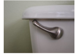
The flush handle can be replaced if it is broken or to improve appearance.
